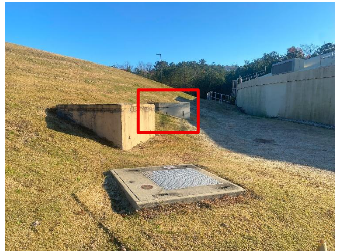
Photo 9 - (SCFP) 96" FW-BFV-5 Clearwell No. 2 Inlet Operator Vault & Surrounding Area
