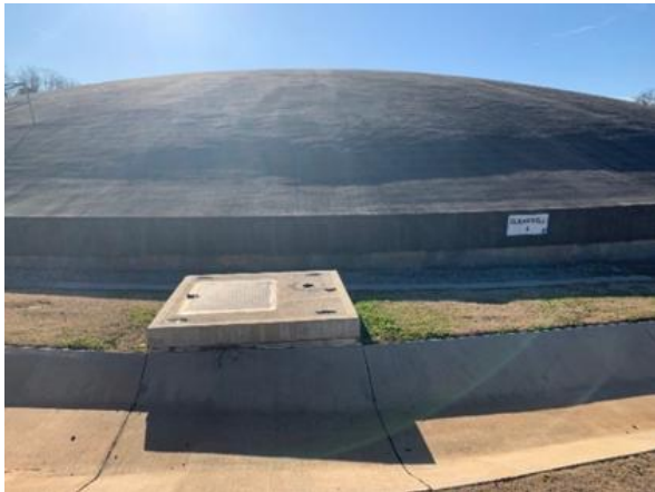
Photo 4 - (LFP) 108" Influent Valve Operator Vault on Clearwell No. 4
