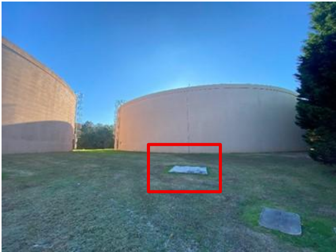
Photo 22 - (SCFP) 54" Valve Operator Vault for RW Equalization Tank No. 2 Inlet (RW-BFV-8)
