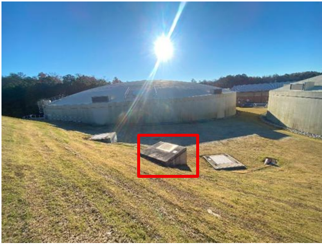
Photo 8 - (SCFP) 96" FW-BFV-3 Operator Vault & Surrounding Area
