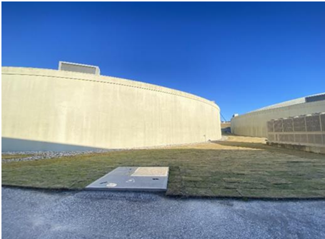
Photo 11 - (SCFP) 108" FW-BFV-8 Clearwell Outlet Crossover Valve Operator Vault & Surrounding Area
