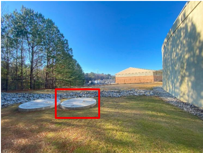
Photo 10 - (SCFP) 108" FW-BFV-7 Clearwell No. 2 Outlet Valve Operator Vault & Surrounding Area
